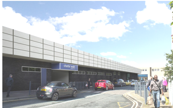
Bankfield elevation - after
